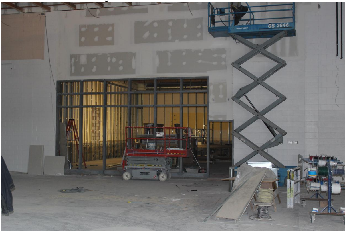
Gym work continues with the framing of the exercise room
