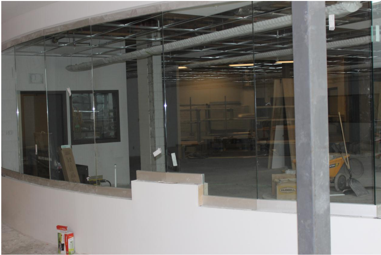
Multi media room and installation of the glass wall
