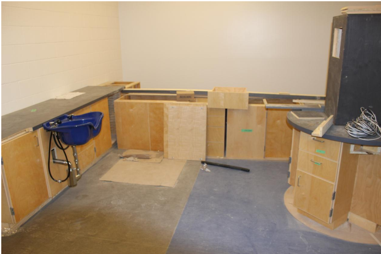
Installation of cosmetology hair wash stations and pedestals
