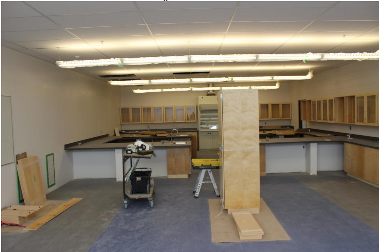
Near completion of the science rooms
