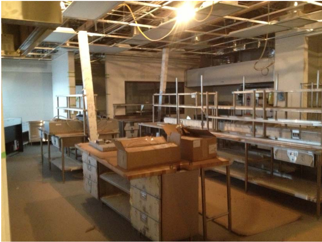
Commercial Kitchen equipment being put into place
