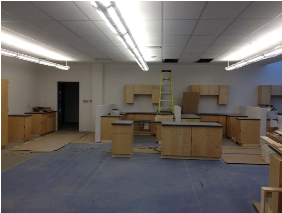
Millwork being installed in the home economics room
