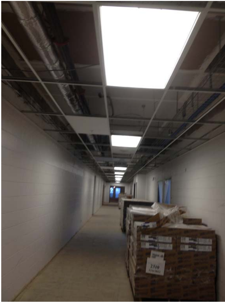
Hallway ceiling grid installation
