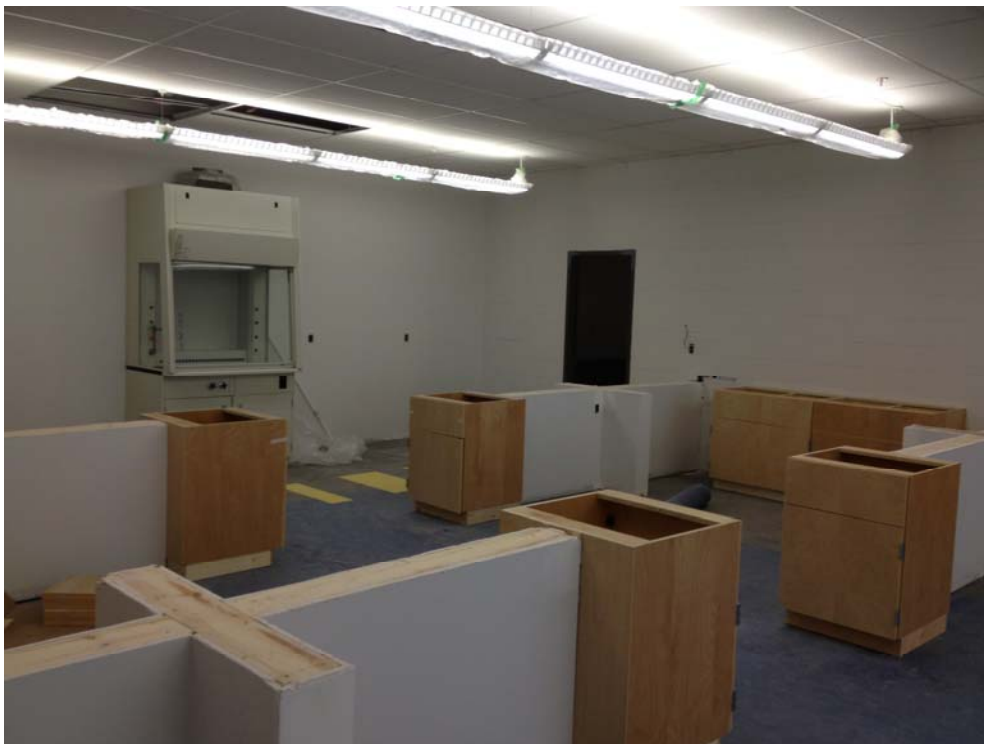
Science Lab fume hood and millwork being installed
