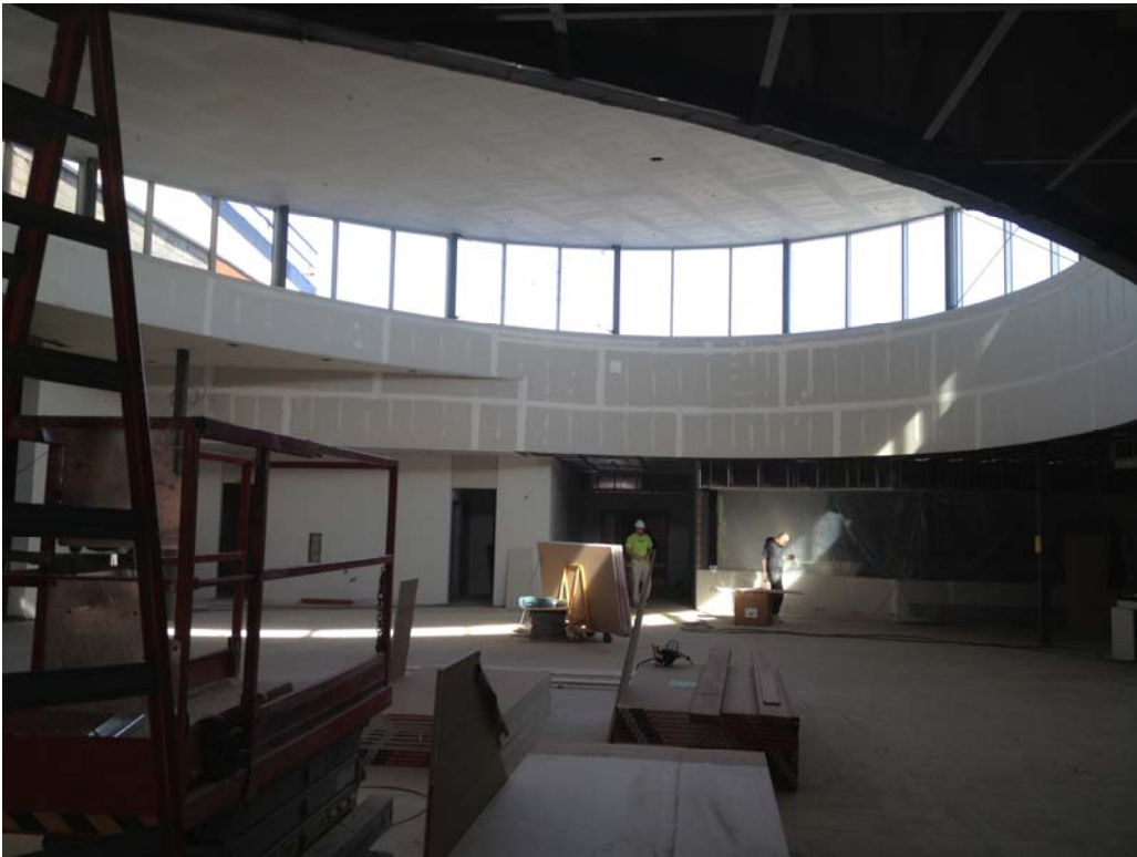
Drywalling and taping completed on common area ellipse
