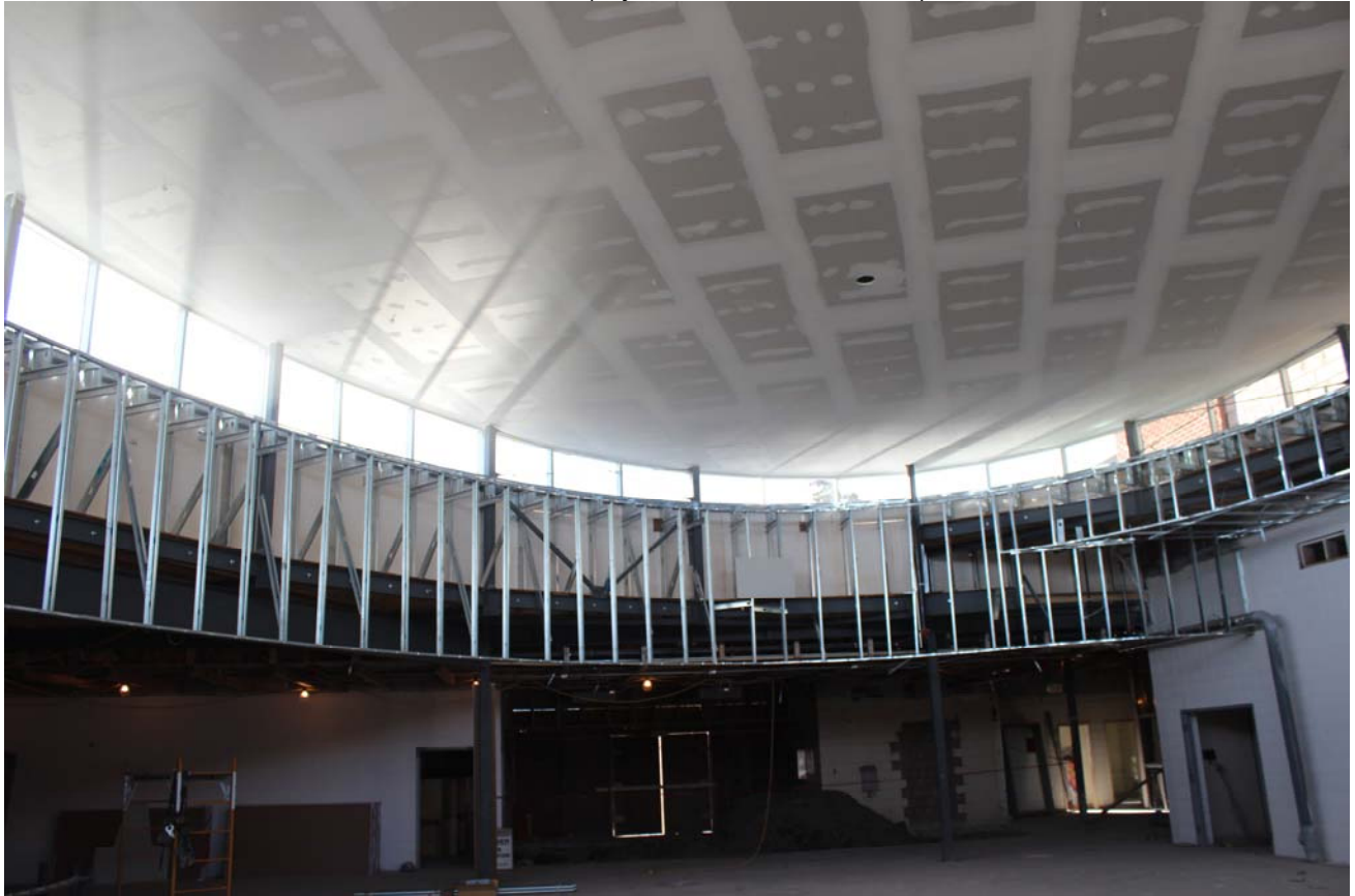
Ellipse ceiling drywalled and taped
