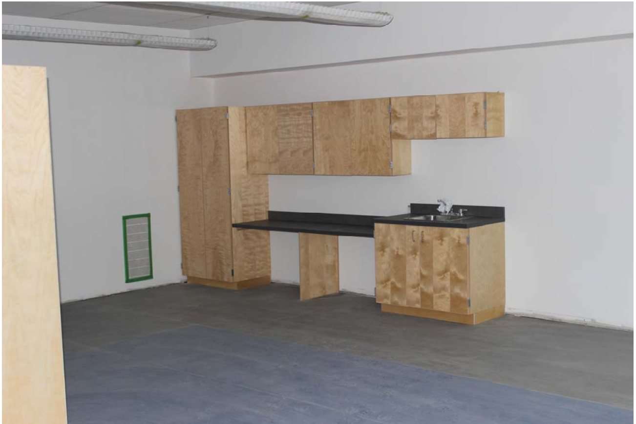
Installation of millwork in a classroom
