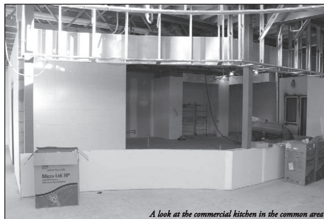
A look at the commercial kitchen in the common area
