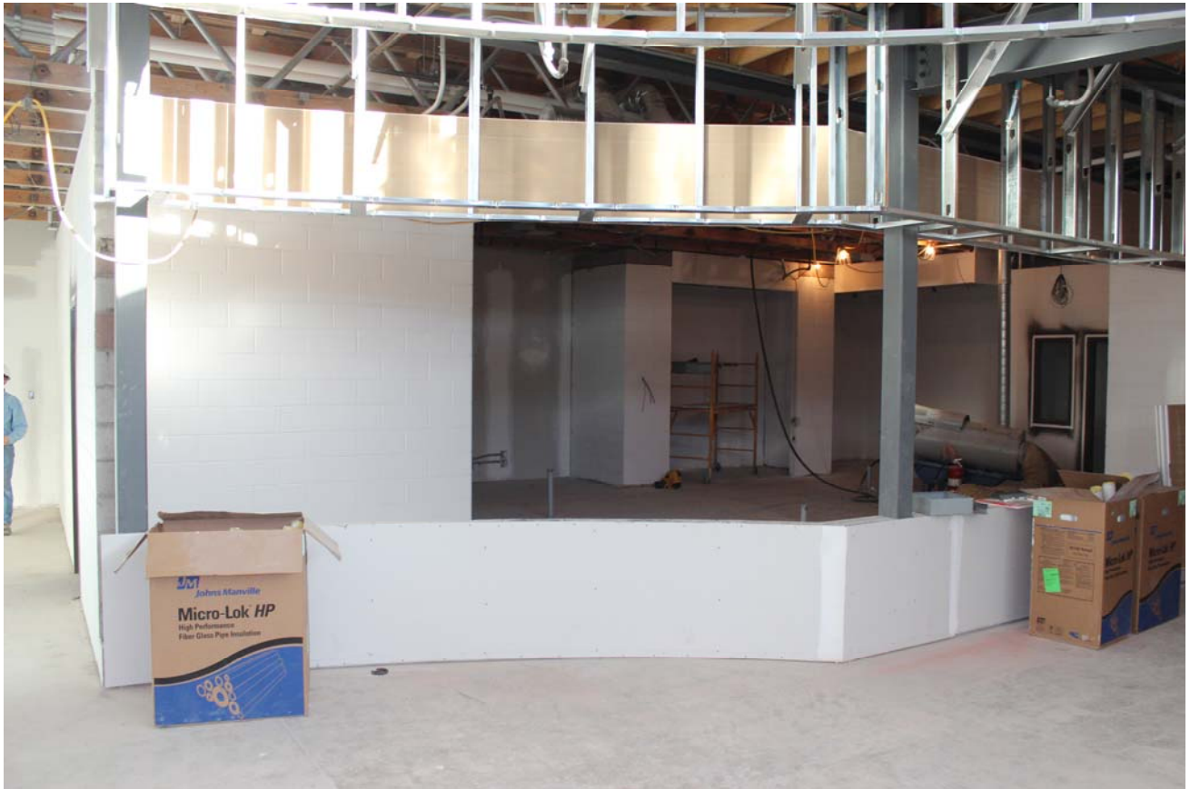
View of the front of the commercial kitchen (drywall has commenced)
