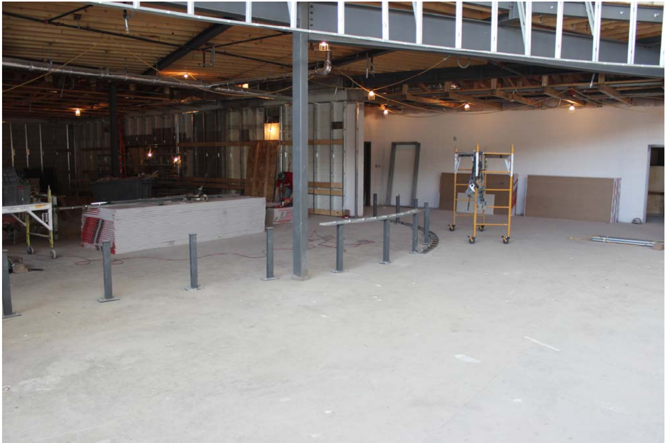
Steel supports are in place for multi media room
