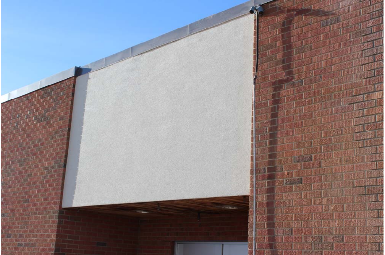
New stucco installation above the east doors
