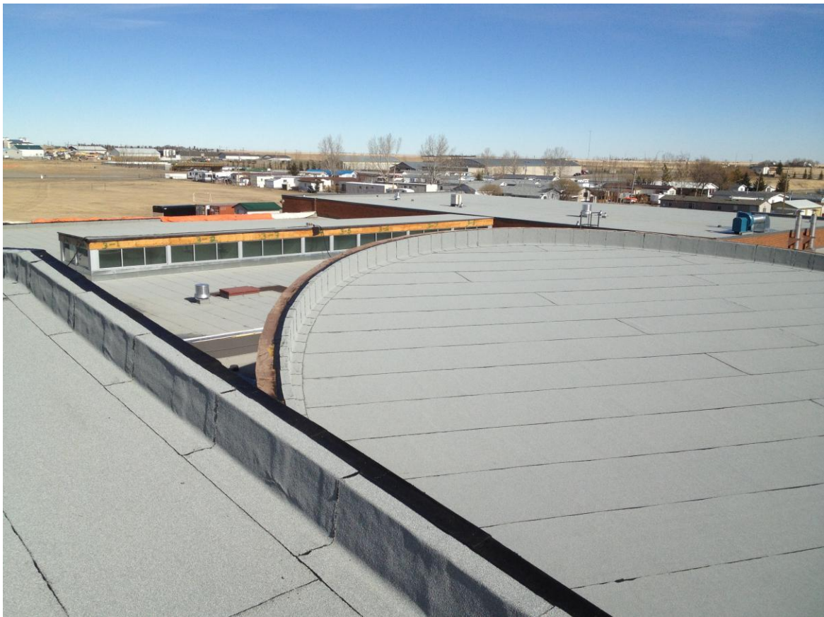
Roofing is completed. Cap Flashing and fascia work remains
