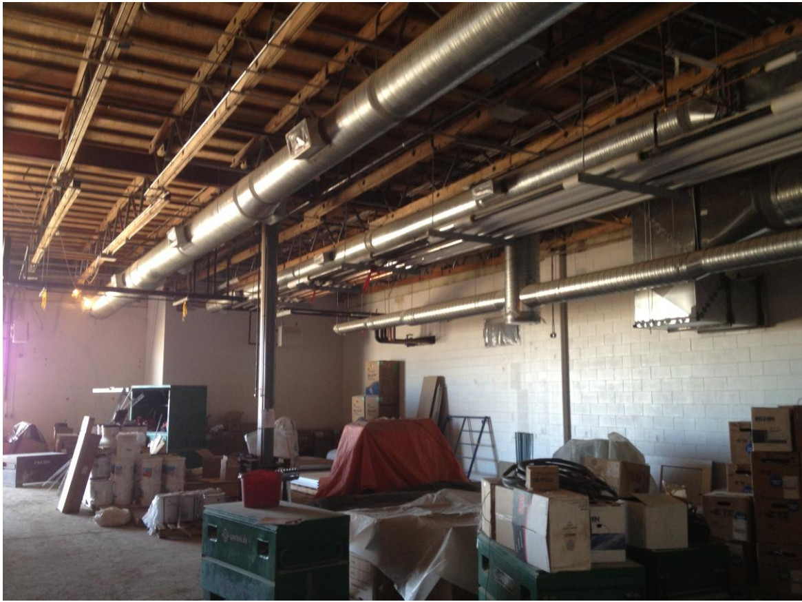
Mechanical installations ongoing in CTS areas
