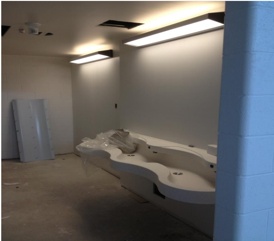
Lighting and lavatories install in washrooms
