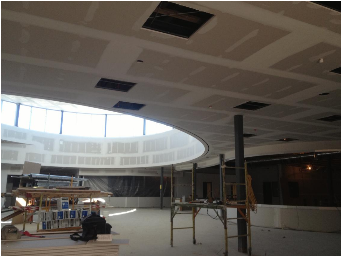
Common area completely drywalled and taped
