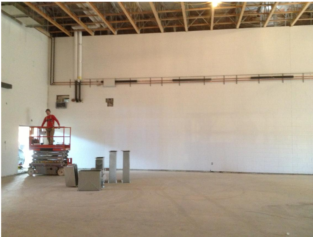
Gym walls have been painted and heating lines are being installed
