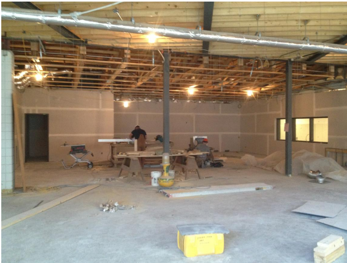
Multi Media area has been drywalled and taping is underway
