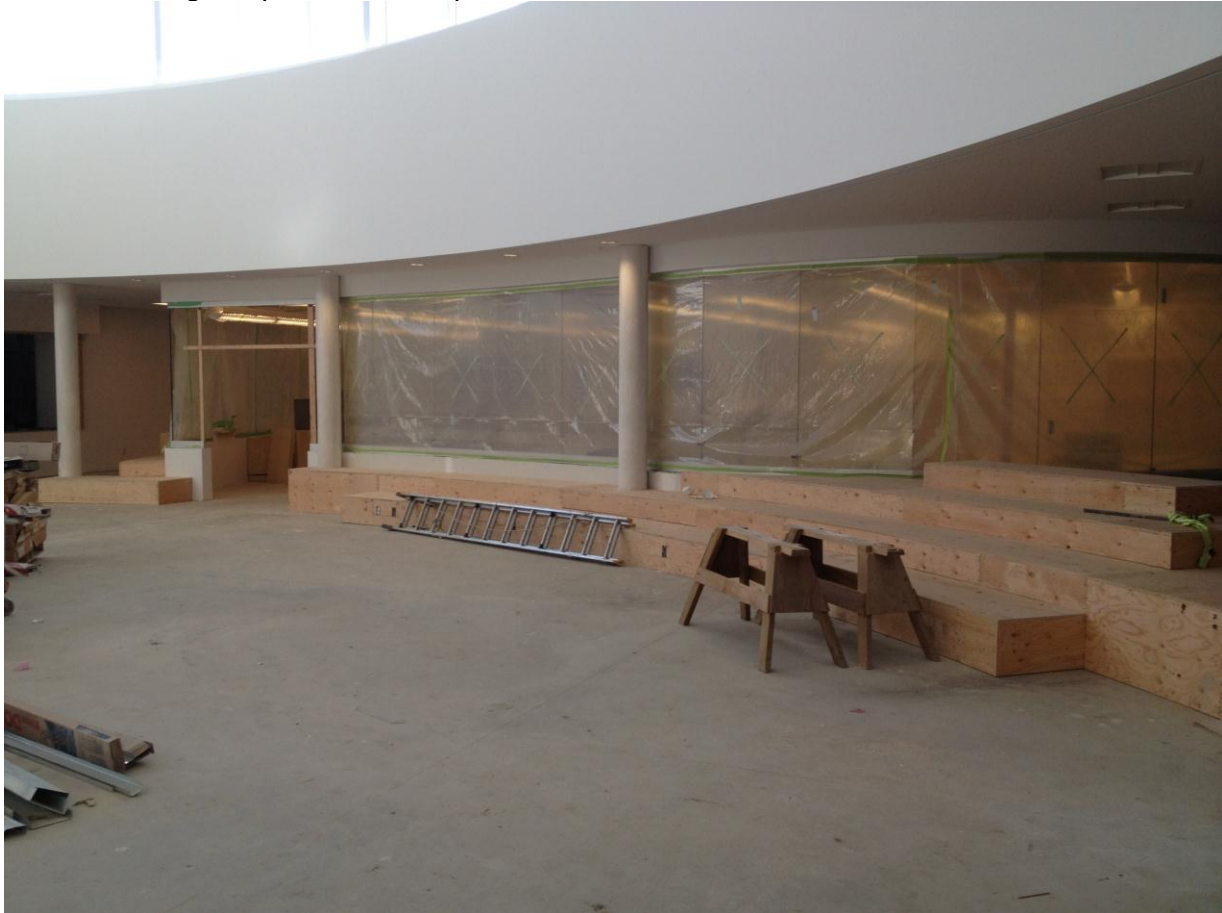
Common area riser benches framed and steel support columns covered
