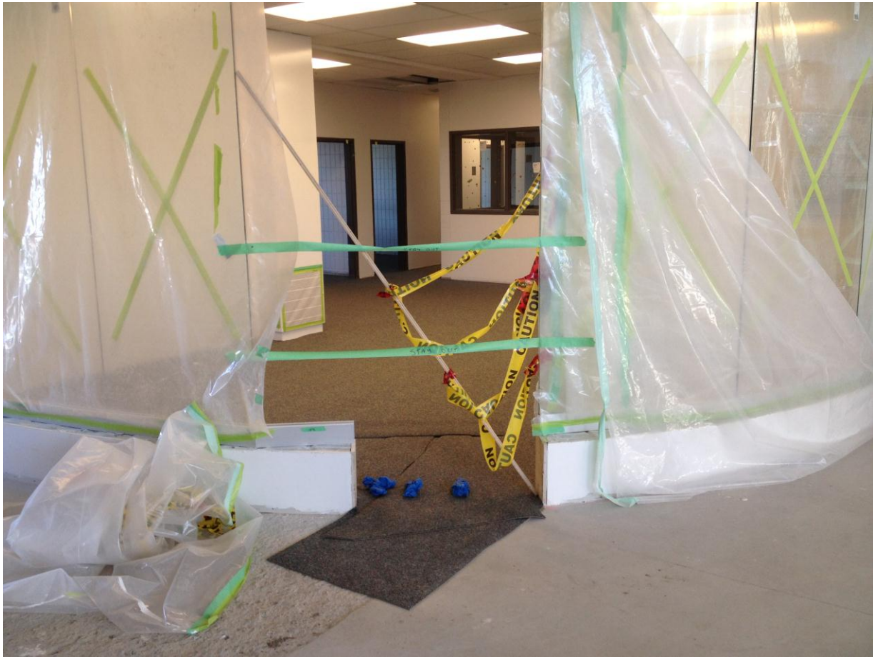
Installation of glass panels and carpet in admin suites
