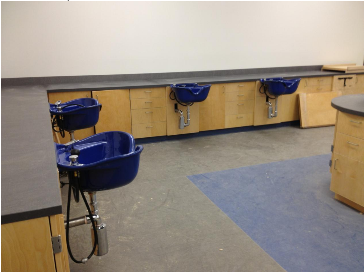
Millwork completed in beauty culture room
