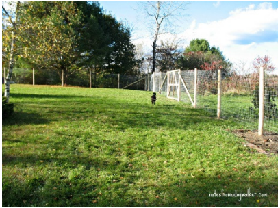
Dog fence Great Falls off leash Dog Park. A wooden square fence post with wire medium to heavy gauge wire mesh stapled to posts
