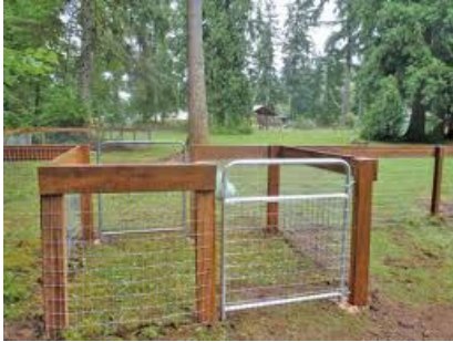
Kalamazoo County Dog Park Fence. T posts with link metal wire fencing.
