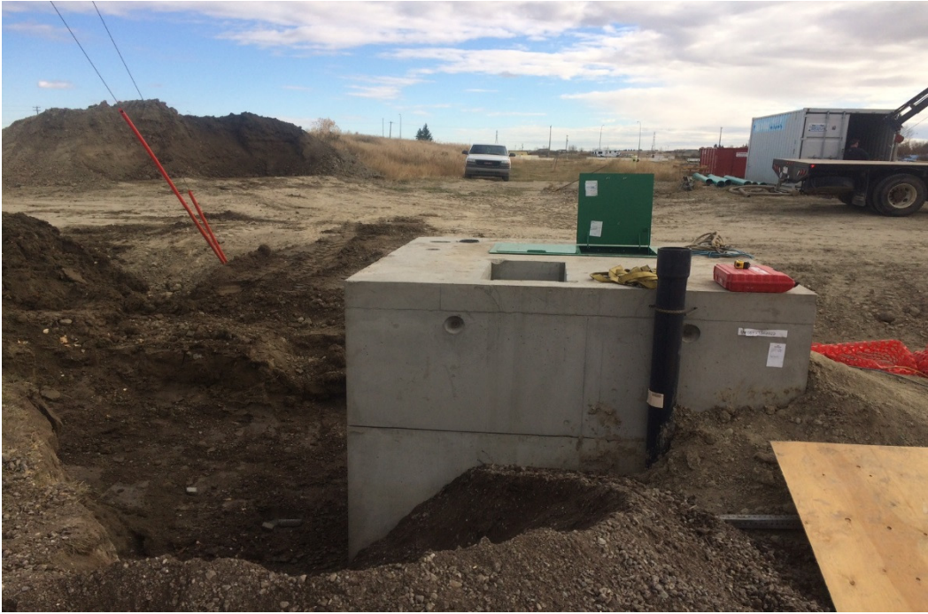
- Harvest Square lift station wet well back filled.
