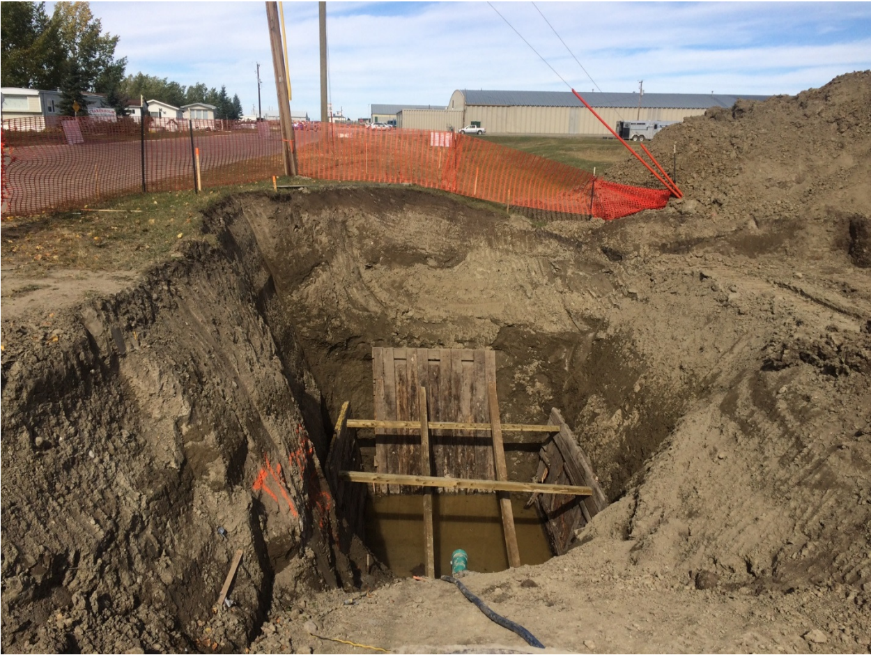
Slurry slab in place to hold the new wet well.
