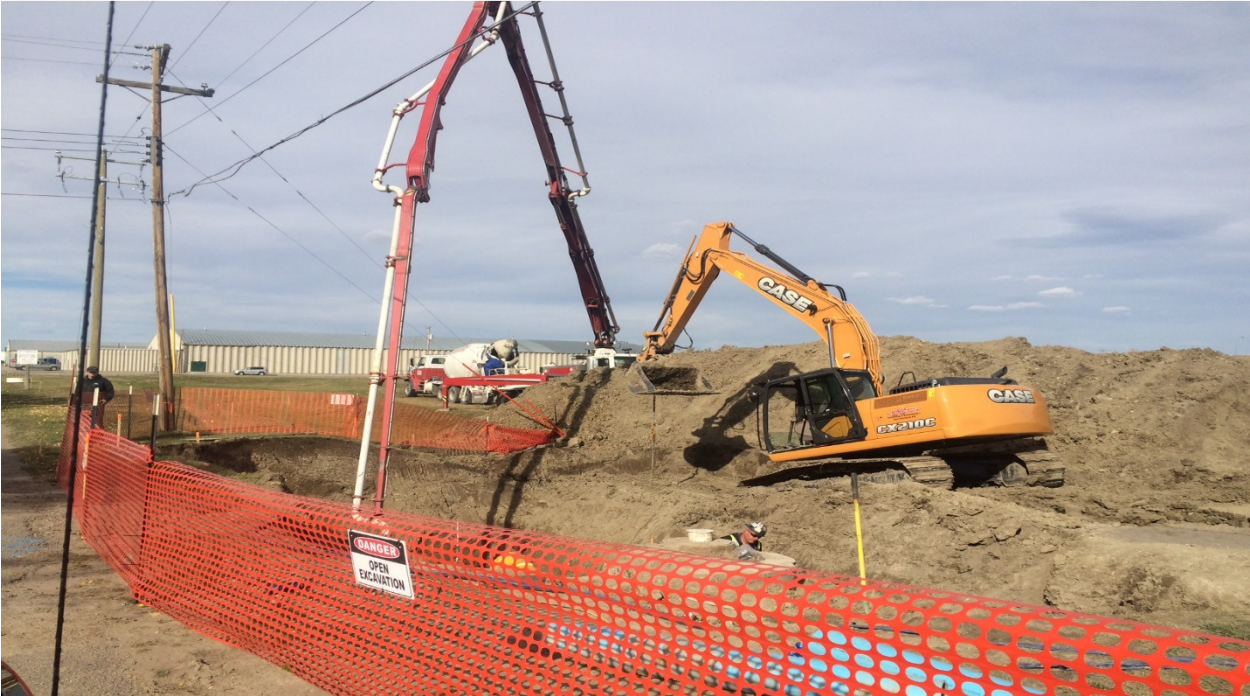
Concrete slurry mixture being pump into the new wet well location.
