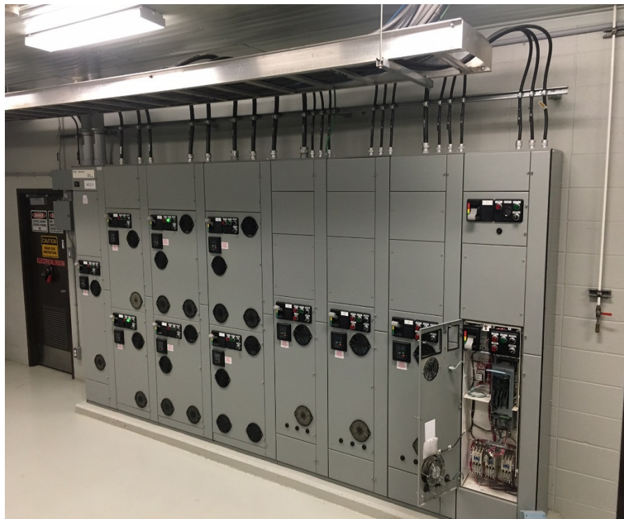
Master Control Cabinet # 4 Containing VFD (Variable Frequency Drives)
