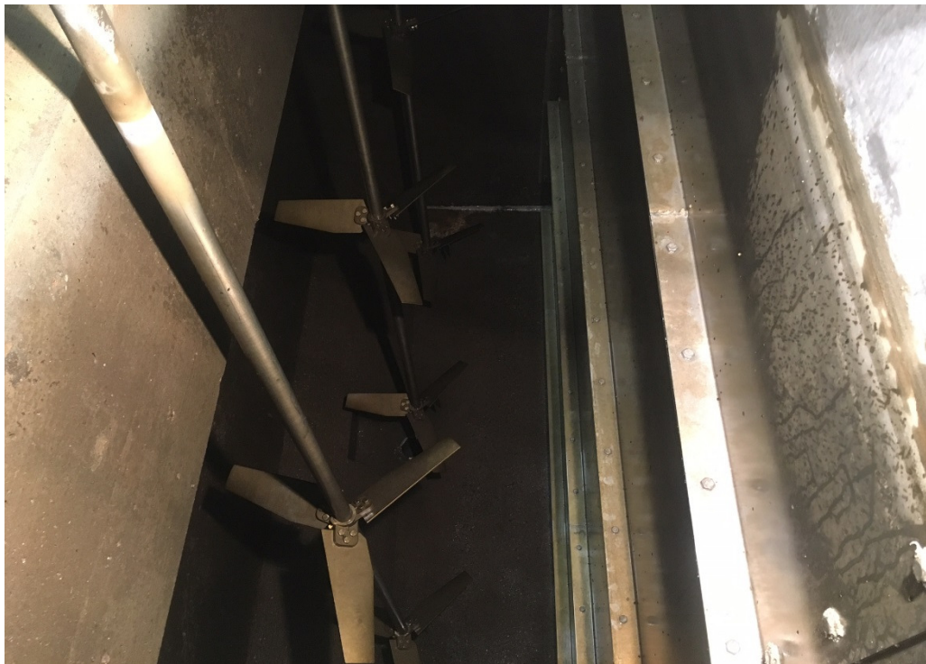
Flocculation Fan Blades Ensures the Proper Mixing of Coagulant for treatment
