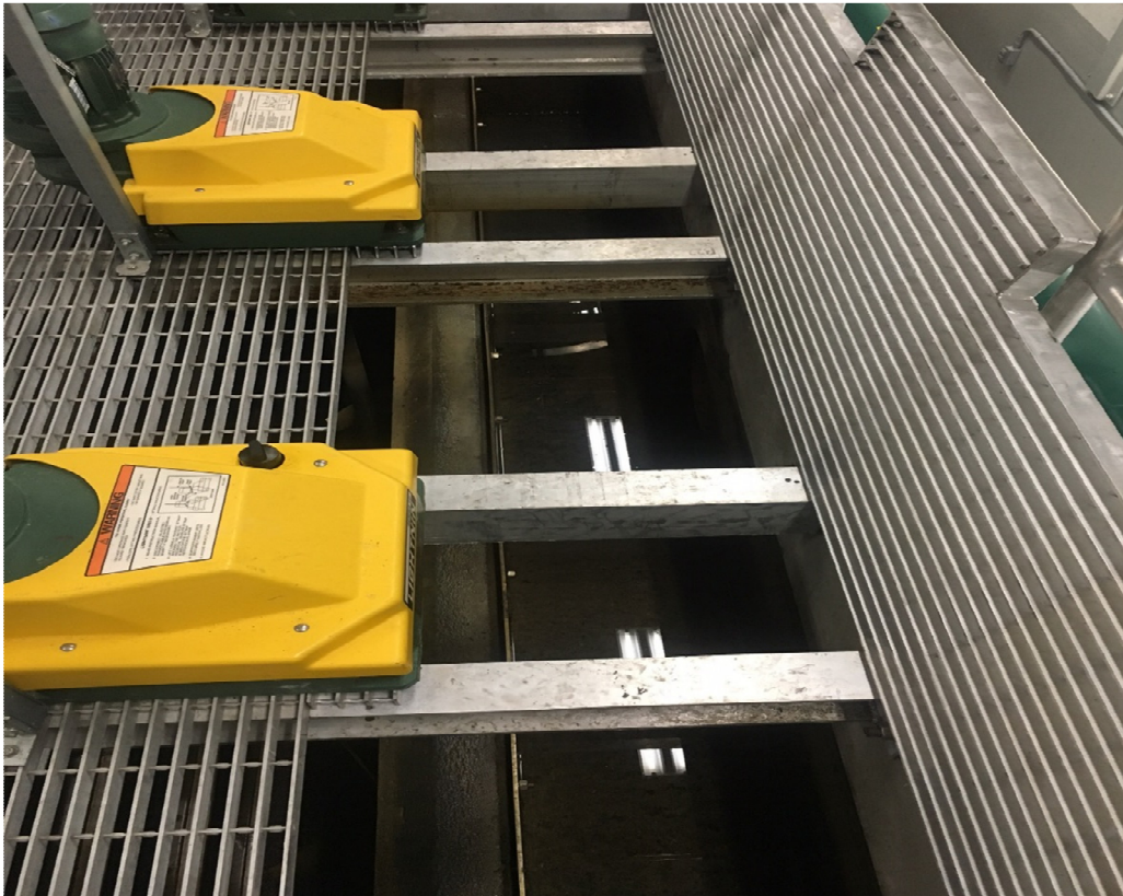
Flocculation Fan Blades Ensures the Proper Mixing of Coagulant for treatment
