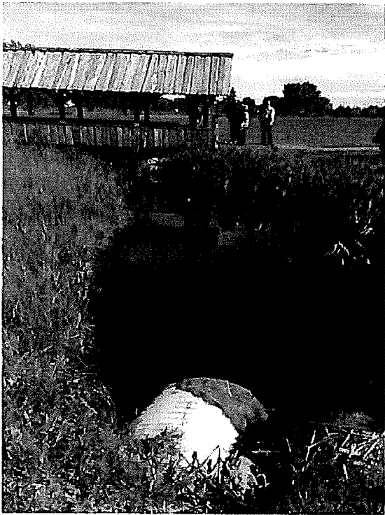
Site Photo 4: Existing old bridge and 375 CSP culverts combined view (photo 1 & 3) Page 2 of 3
