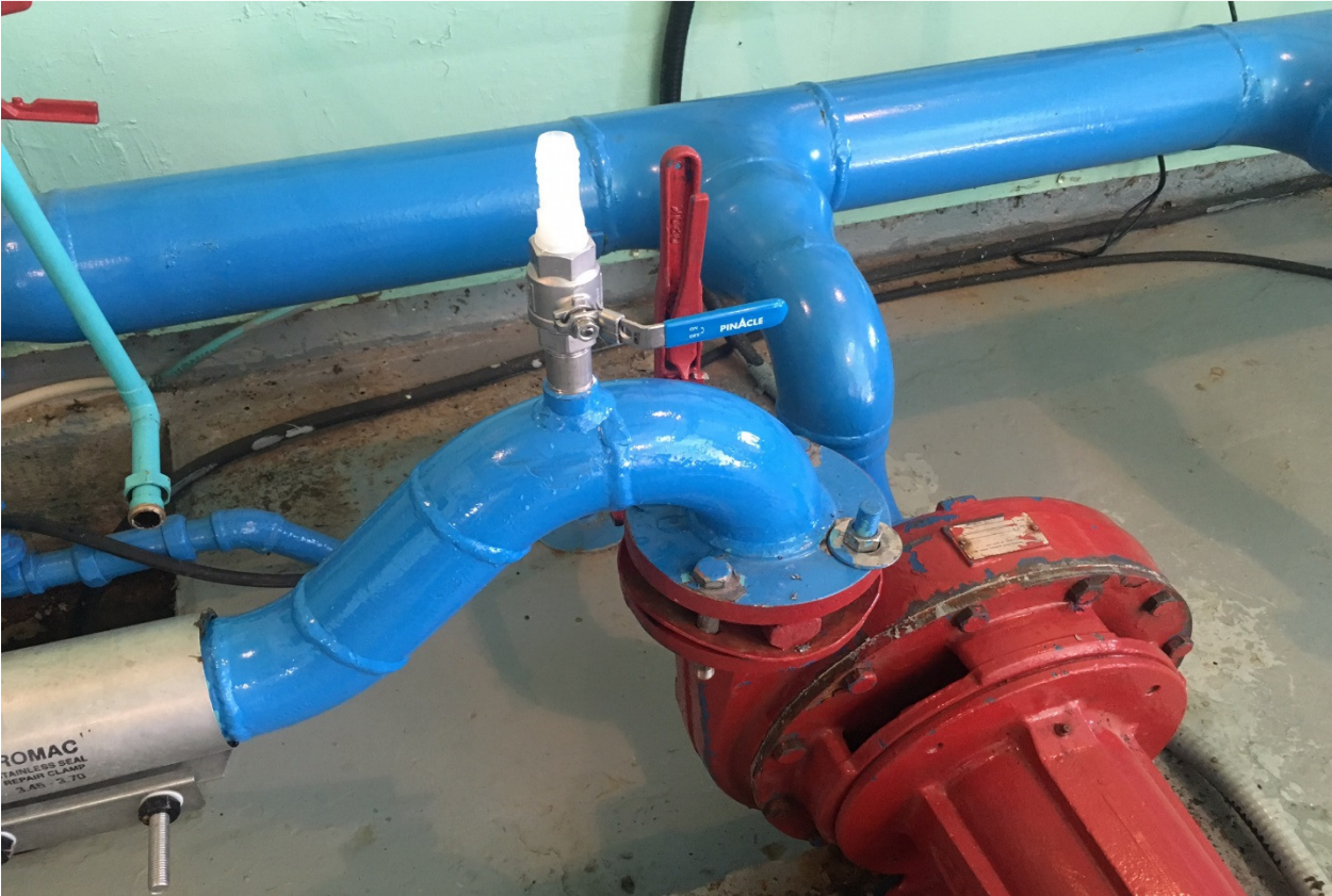
Air Suction Port Installed at the Airport Pump Station and Recently Replaced Distribution Pump.
