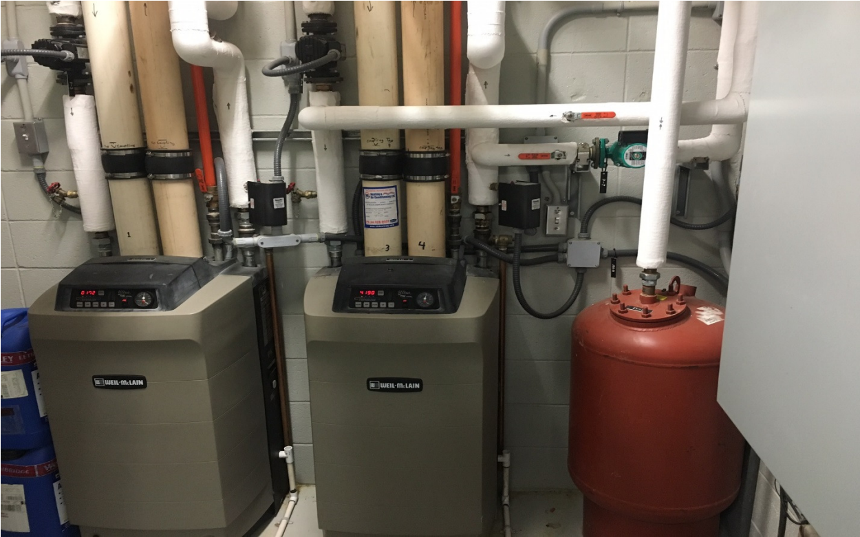
Domestic Hot Water Pump P-7 Replaced In Mechanical Room.
