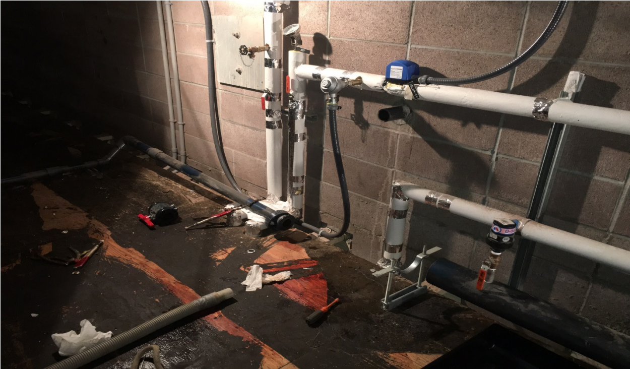
Air Suction Port Installed at the Airport Pump Station and Recently Replaced Distribution Pump.
