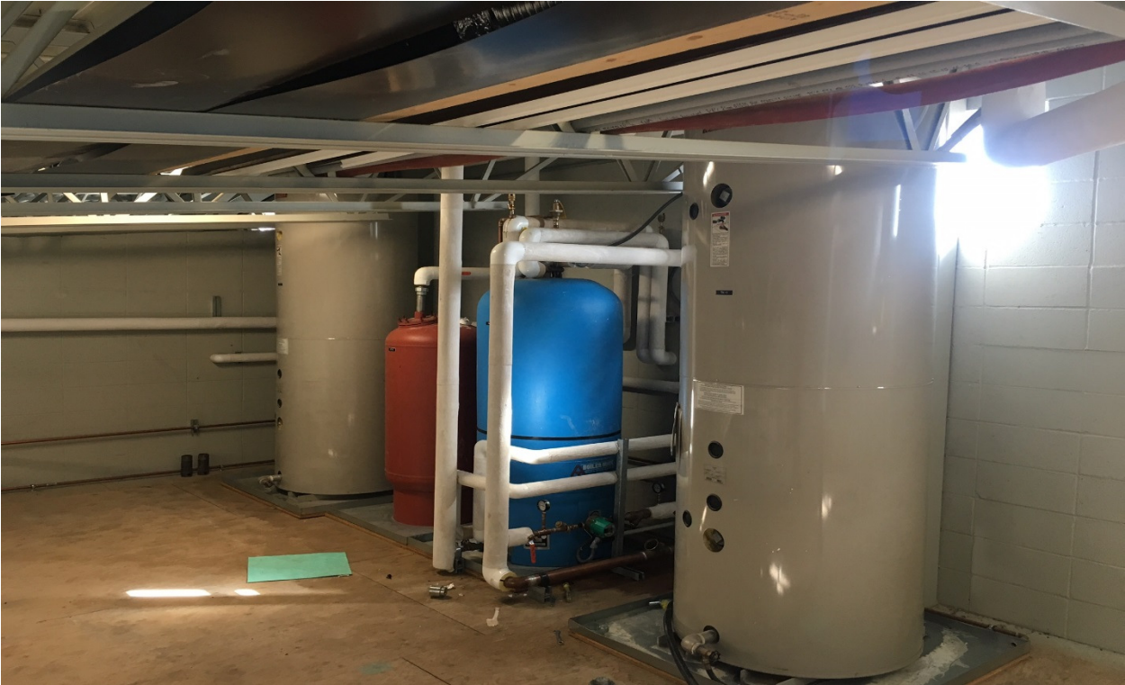
Space above the Distribution Area Containing DHW and Solar Hydronic System Piping.
