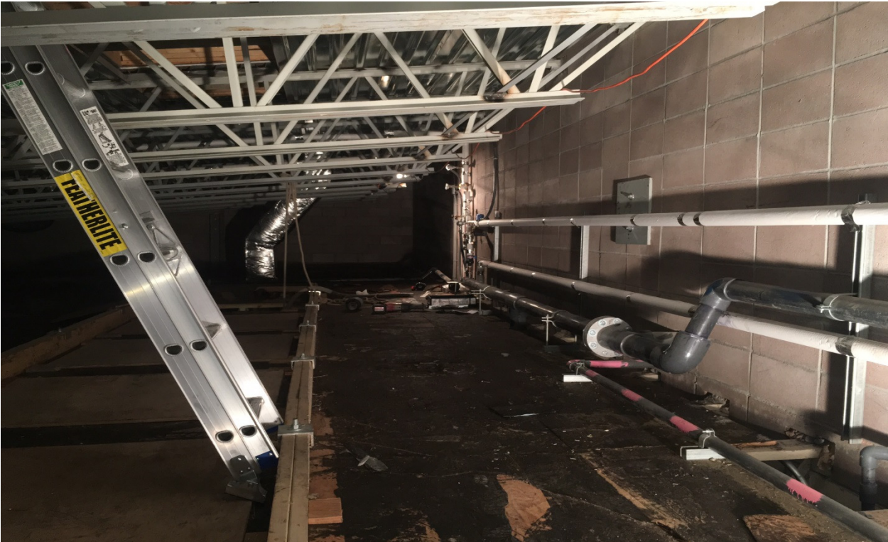
Space above the Distribution Area Containing DHW and Solar Hydronic System Piping.
