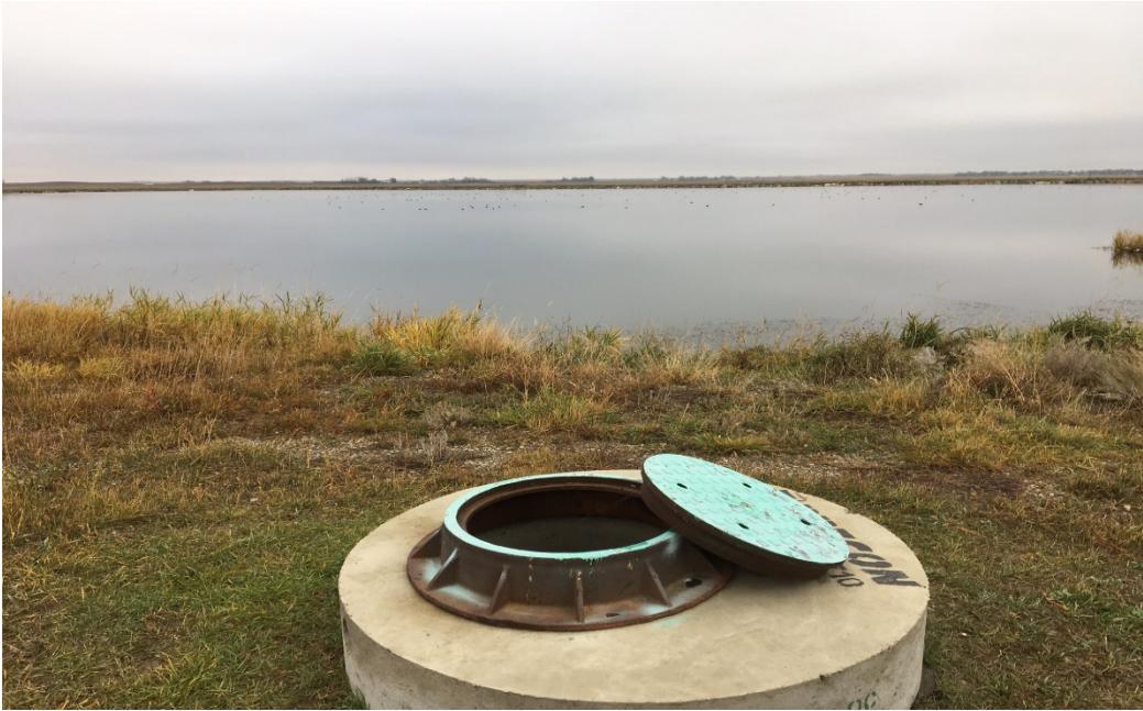
Wastewater flow from clear water holding cells
