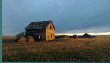
Abandoned farm buildings southeast of Granum
