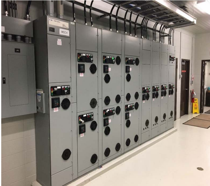
Master Control Cabinet (MCC) #4 Contains 11 of 23 WTP VFD's
