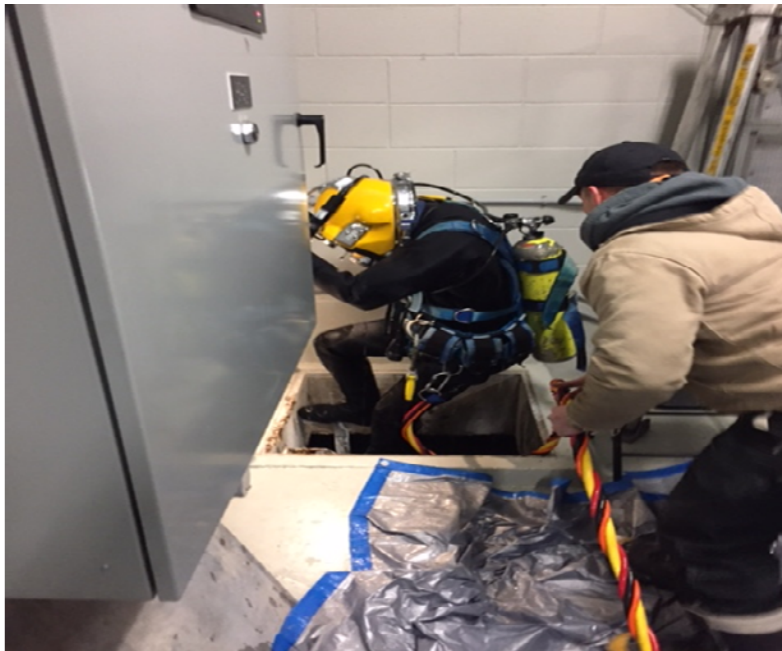
Diver entering North West hatch inside HPS building
