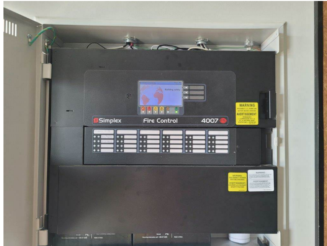
Photo #10: Fire alarm panel
