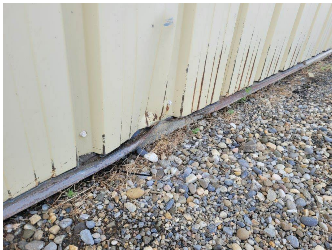
Photo #6: Typical corrosion at west elevation
