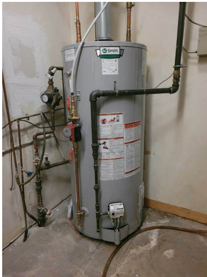
Photo #19: Main Hall hot water tank heater
