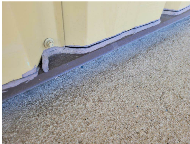
Photo #5: Sealant deterioration
