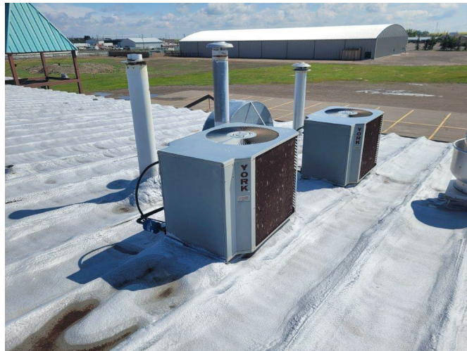
Photo #17: Typical condensing units
