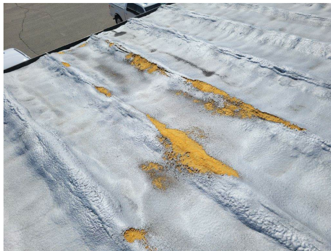
Photo #8: Typical deterioration on sprayfoam coating
